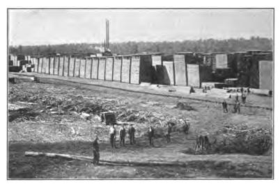
Fig. 92.—Lumber yard of a sawmill in the Lake States. Note fine appearance of lumber piles. The discarded material in the foreground is, however, a dangerous source of infection and should be burned.
